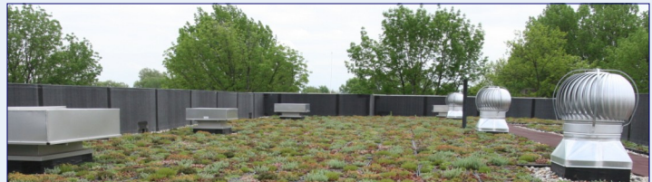
The Green Roof at Nellie Reynolds Gardens in Philadelphia.
